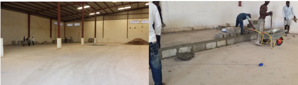
The beginning of partition wall construction in Ghana
